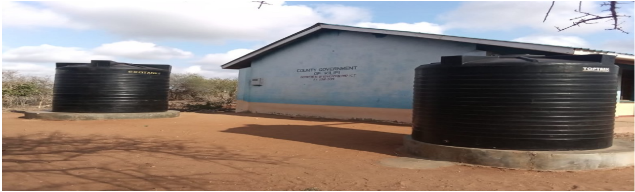
The two other tanks.
